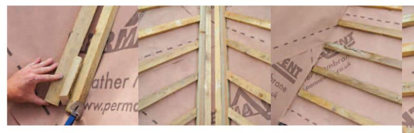
(There should not be more than 20mm gap between the wall and the end rafter. With a large gap the membrane can gradually fall down this gap and should therefore be supported or fixed to the abutment using the double sided tape).
