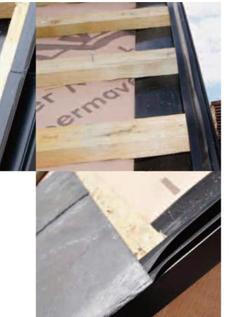
Easy Valley should be 'v' cut and positioned to allow the rainwater to flow into the guttering.
