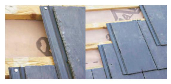
Dry ridge and hip systems must be used at lower pitches. The ridge roll should be fully stuck to the hip/ridge slate using the tape that is applied to underside of the ridge roll. Cover flashings at wall and abutments should be fixed in place using double sided butyl tape. Top flashing should extend at least 200mm down the top slate on low pitches. The side lap of the top flashing should also be sealed on a low pitch.
